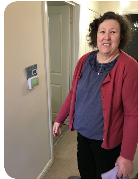
A Flagship resident with her new switchee freshly installed
