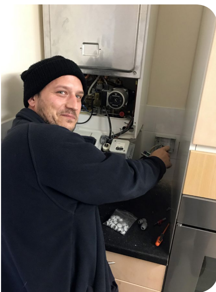
A Flagship installer fitting the Switchee boiler controller
